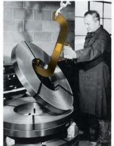
With the hook in place, the wedge pivots as the lift is started, and the coil begins to turn to a vertical position for transporting.
